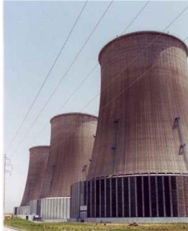
**Photograph of indirect dry condenser cooling system.**
